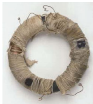
The first transformer 29 August 1831
